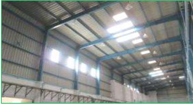
Transparent sheets for roofing at regular intervals
