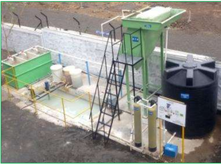
← Effluent Treatment Plant
